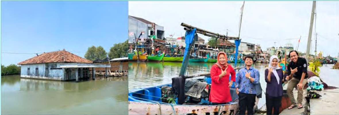
Houses inundated by tidal flooding (rob) and fish landing activities operating under non-flood conditions.
